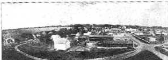
View of the new plant at St. Lawrence, Minn., showing the large open space and the buildings.
