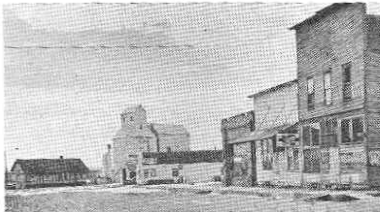
SHERMAN'S MAIN STREET, with several empty buildings, displays only a fraction of the business activity that it did at the turn of the century.
